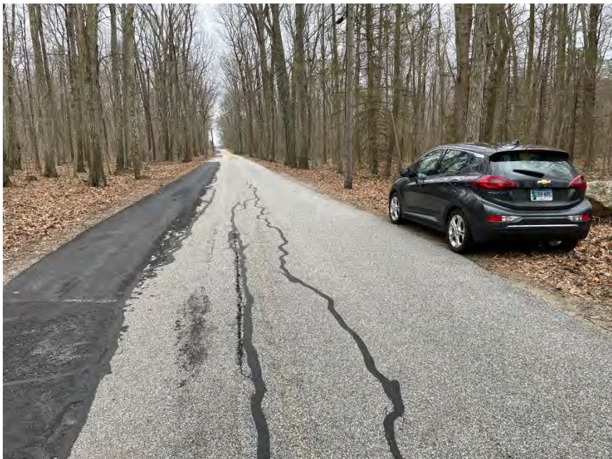
Photo 2: Proposed pulloff parking on Wheeling Road facing south.
