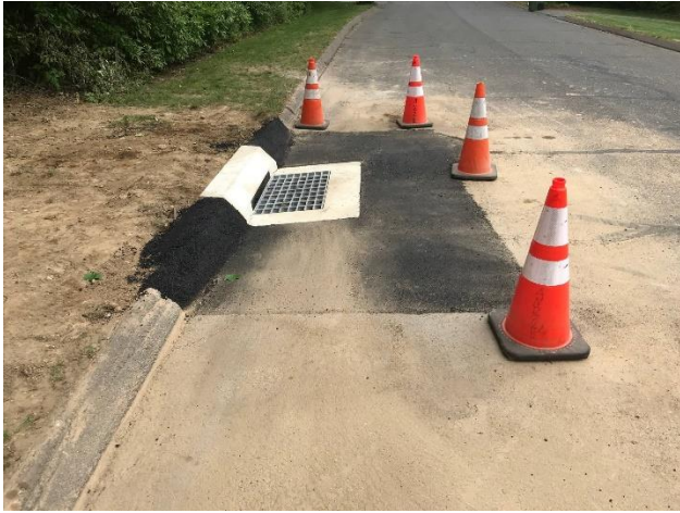
Stanley Drive finished basin
