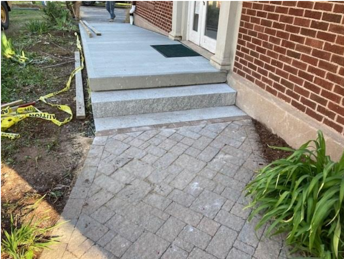
Library walkway and new steps
