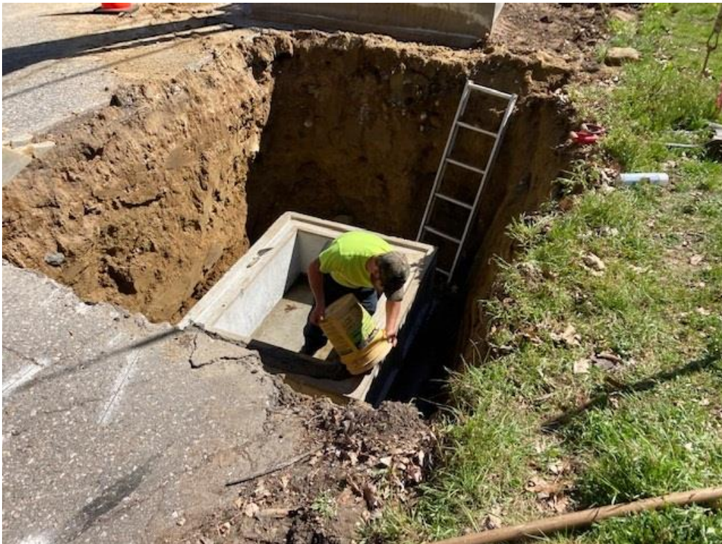
Drainage work on Shoddy Mill Rd Installing new Basin
