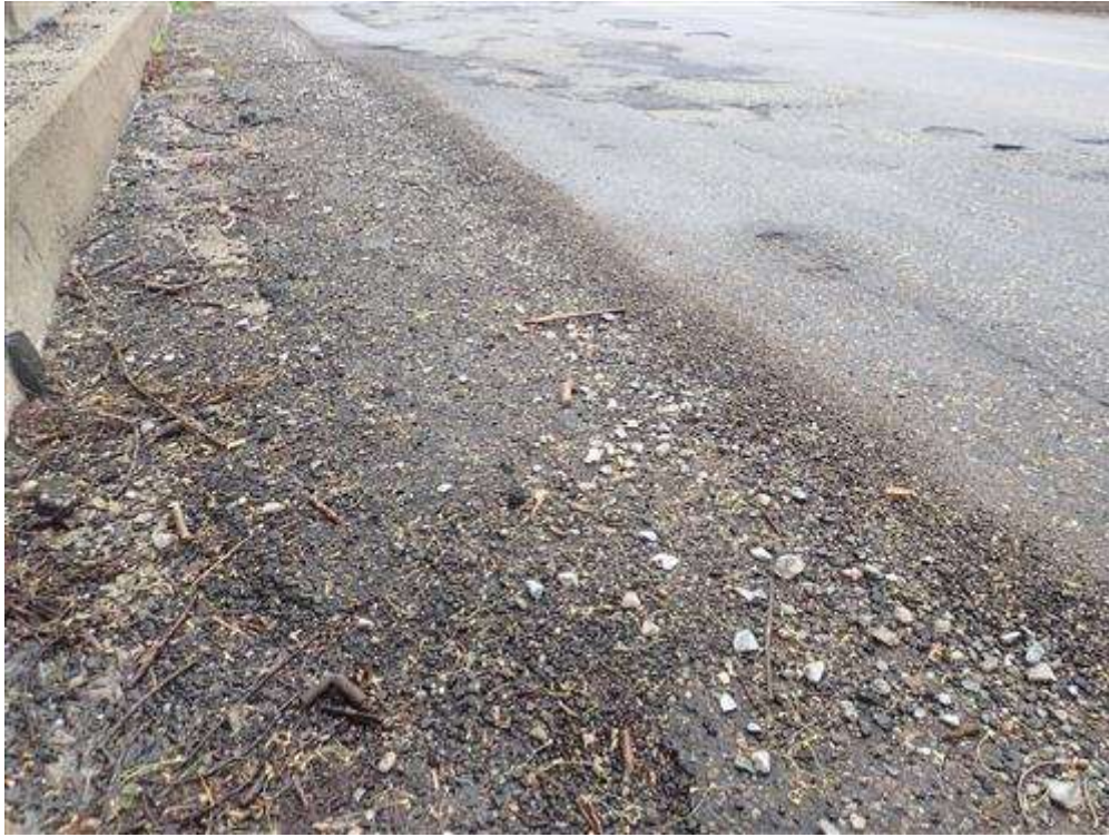
Top of deck exposed full length along east curbline
