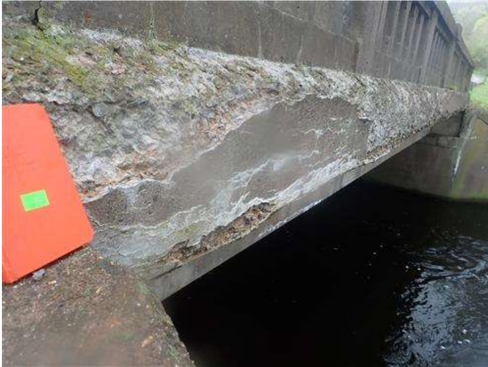
Severe scale along east rail base fascia
