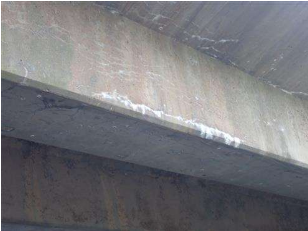
± .012" open cracks along beam 5 fascia
