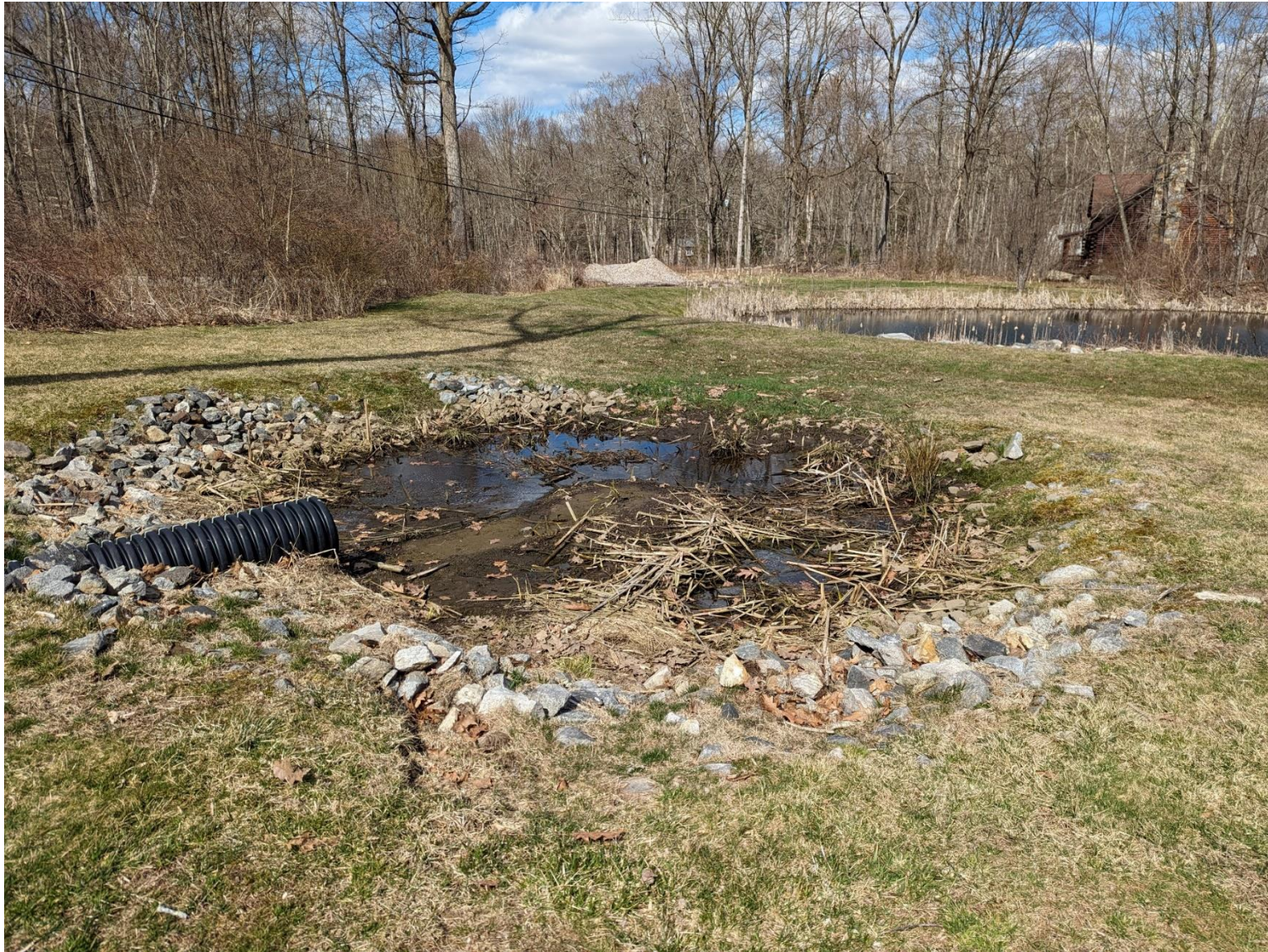
2 - View of plunge pool. The man made pond is in the upper left corner. The pipe in the plunge pool is connected to the open basin near the road. Water flows from the road into this pipe, then under the driveway into this plunge pool.
