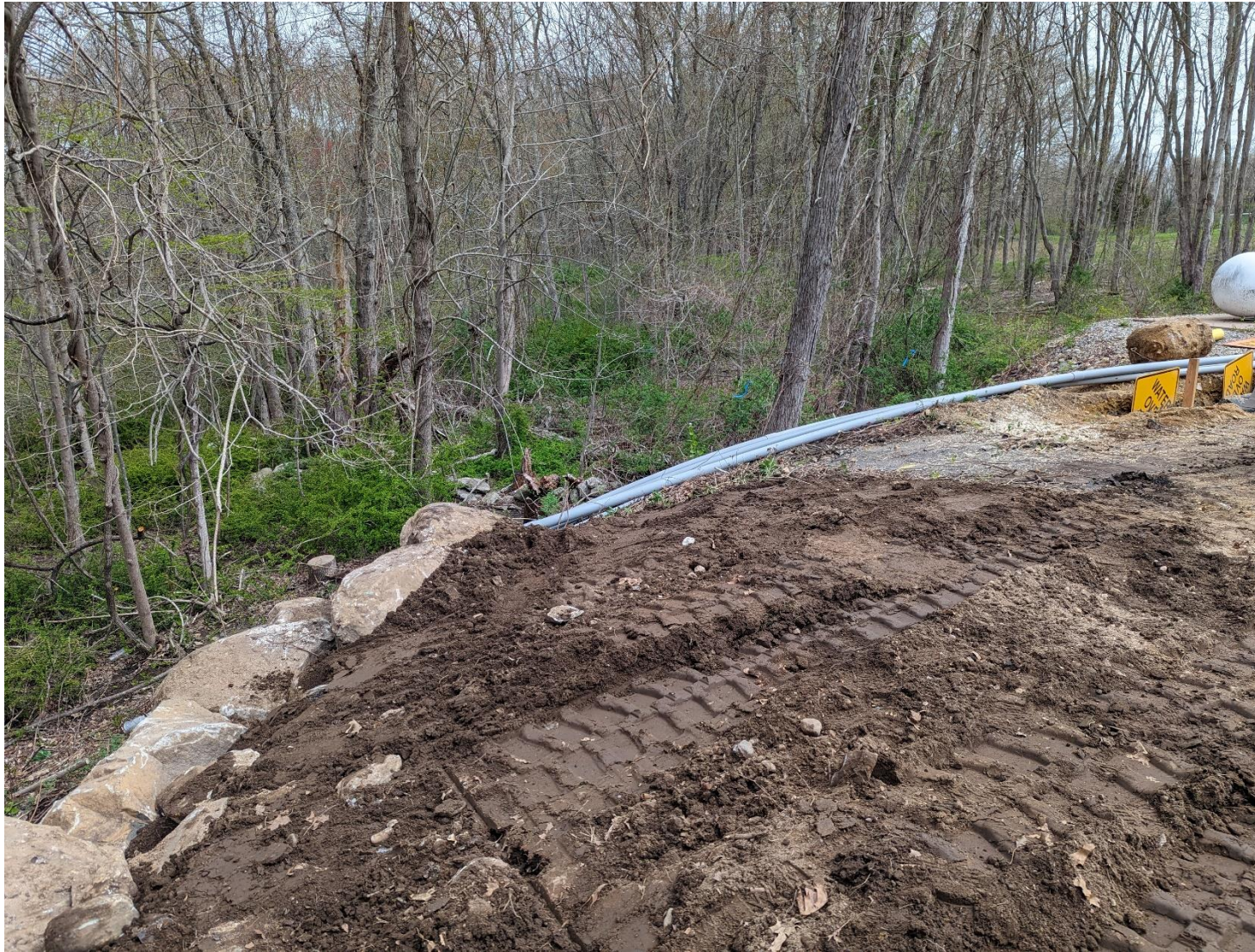
1- View of edge of filled area in URA. Trench will be dig in this area, and area will be stabilized with seed. Wetlands are to the upper center and upper left of photo.
