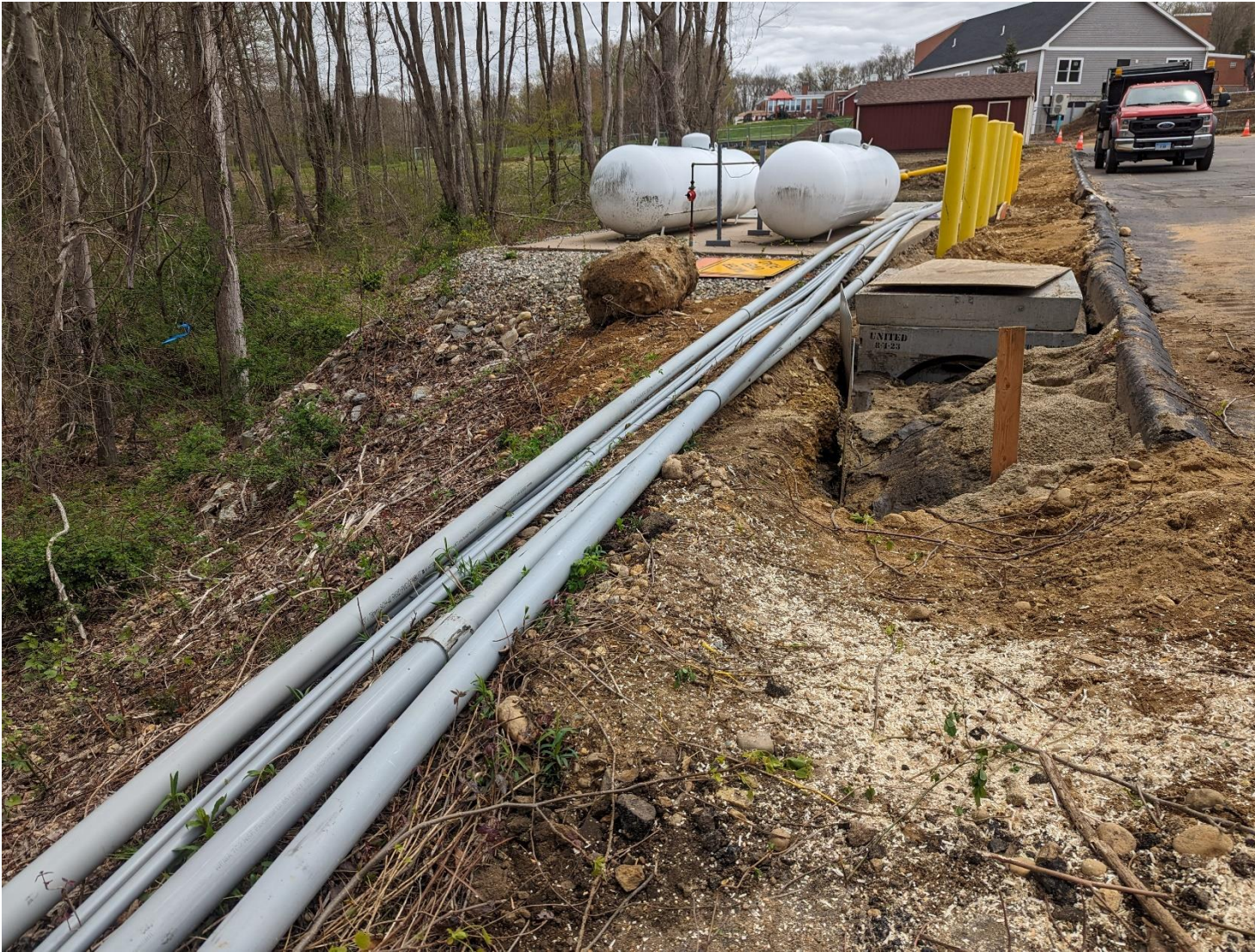
2- View of propane tanks and utilities trench, which will continue through URA and lead to fire station.
