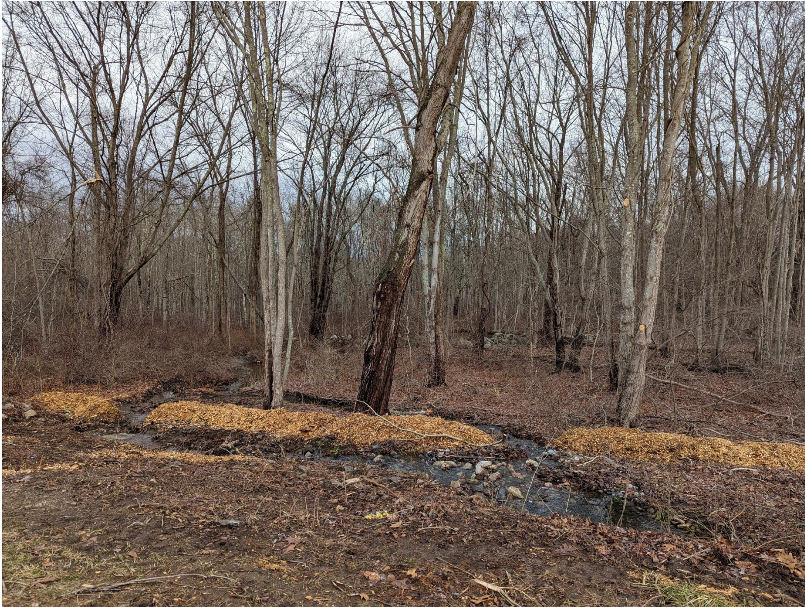
4- View of cleared work area, looking north from the parking lot. Invasive plants in the area have been removed, and vines have been cut or removed (where possible) from trees. Mulch berms have been placed for erosion control during work.
