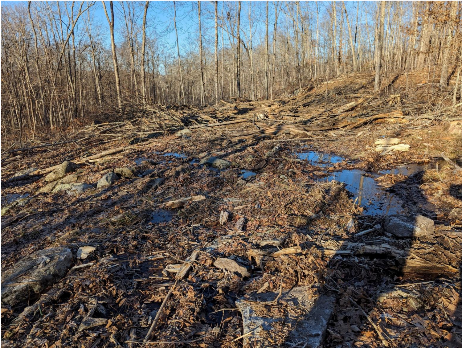
12 - View of wetlands crossing (the second on the map, if counting from south to north). Stream channel was left intact with minimal disturbance from temporary bridge. Tree limbs seen in photo will be left in place to stabilize approaches to the crossing.
