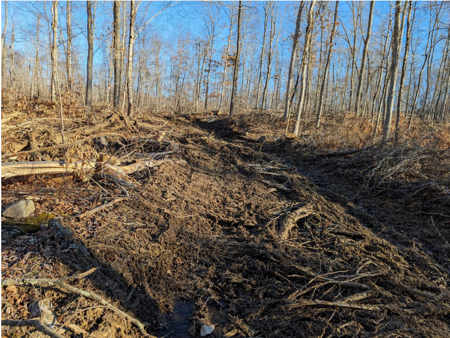
4- Looking north on main skid trail, north of the large southern wetlands crossing. This area is the most rutted area of the trail and is outside the URA. Area will be filled and raked to eliminate the large rut, and will be seeded in the spring.
