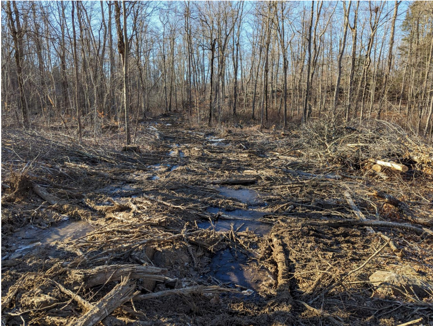
6 - View of approach to wetlands crossing, which is behind me in the photo. Logs and woody debris will remain in trail to stabilize area and limit erosion into the wetland. Exposed soil will be seeded in spring.
