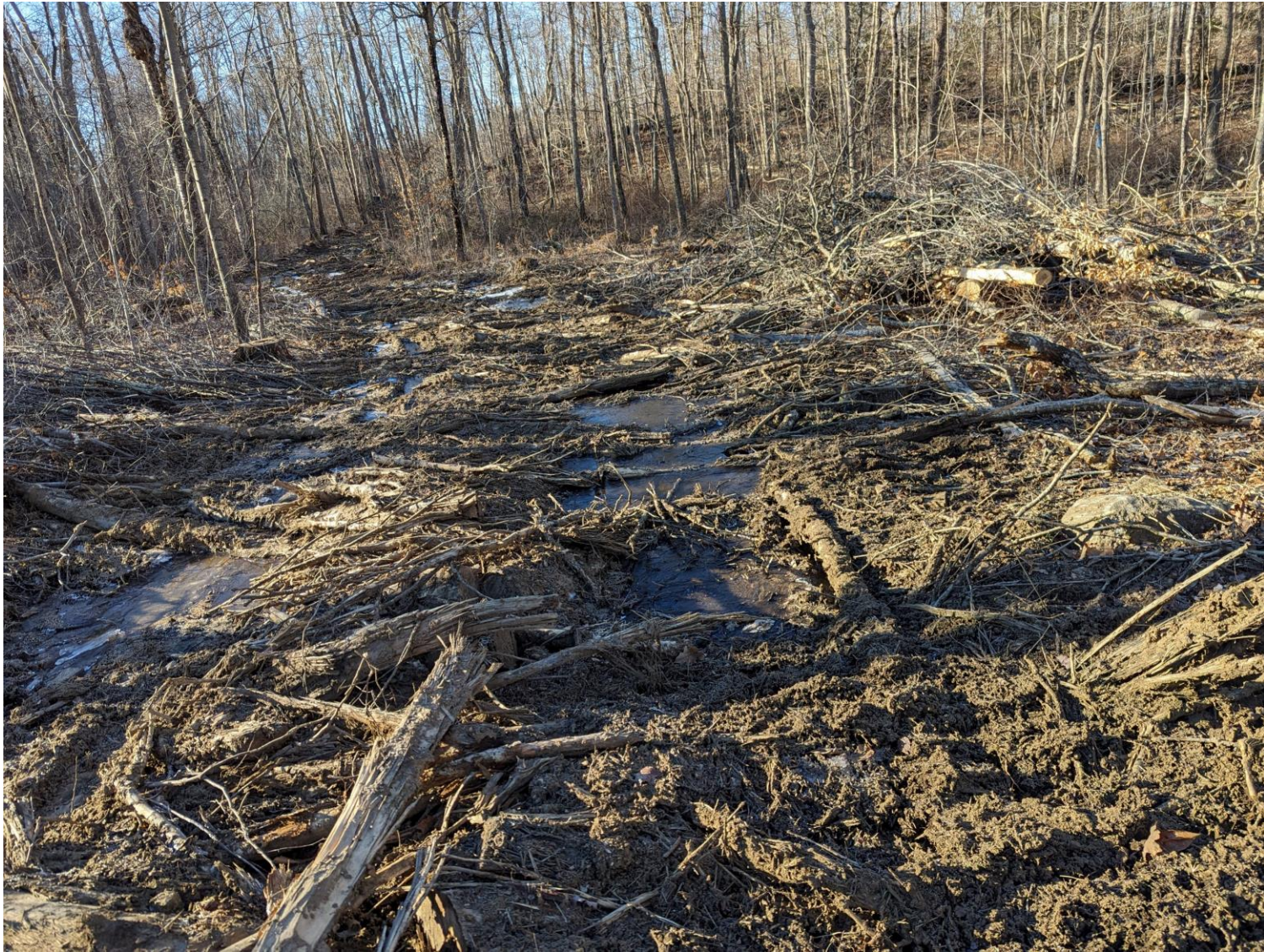
5- View of approach to wetlands crossing, which is behind me in the photo. Logs and woody debris will remain in trail to stabilize area and limit erosion into the wetland. Exposed soil will be seeded in spring.
