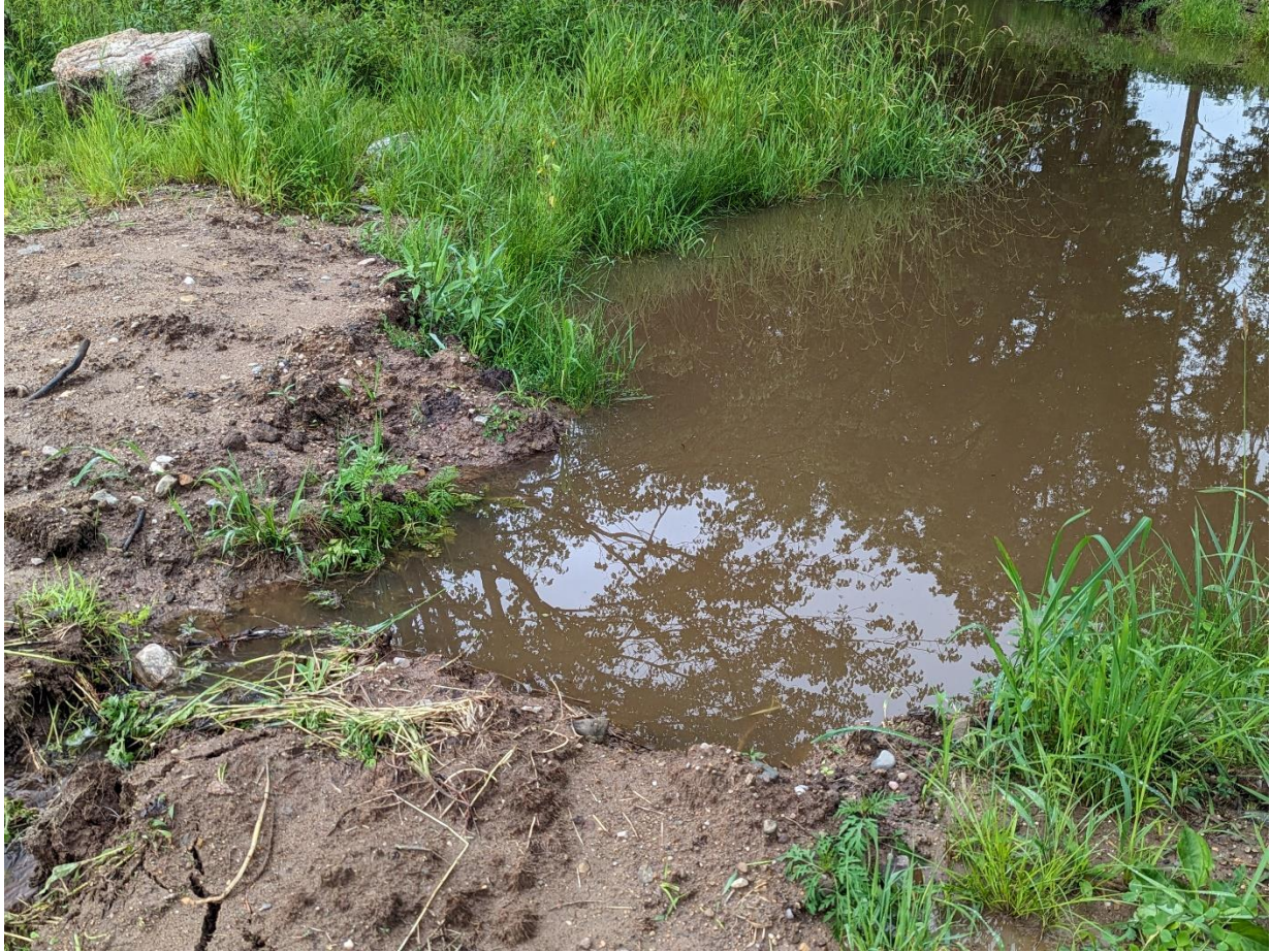
4- View of western edge of pond, near newly constructed (and currently dammed) outlet created by the homeowner. Pond is unable to properly drain through the original outlet and stream, and has started to flow over the temporary dam.
