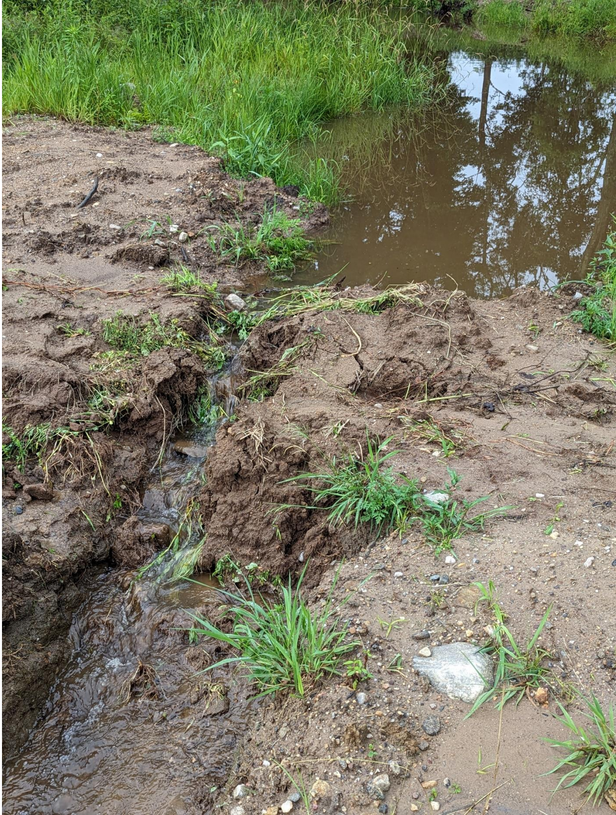
5- Another view of the breached temporary dam at the western edge of the pond. Homeowner has since repaired the dam and extended it by filling more of the downstream channel with rocks and soil.
