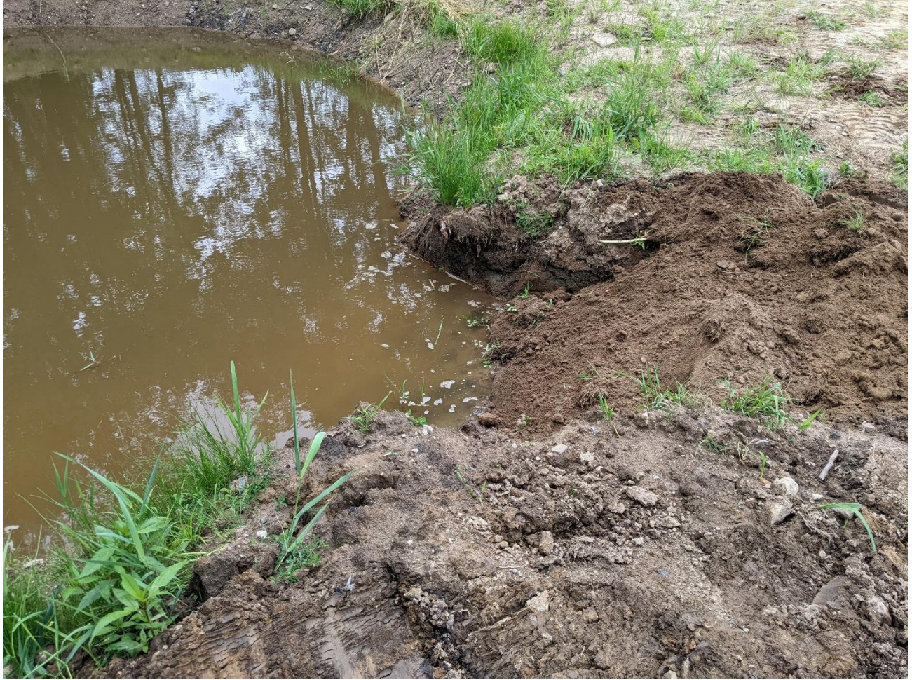
16- View of new pond outlet created by owner. This was taken during placement of of rocks and fill to create a dam and to redirect the water into the existing stream until a permit application can be reviewed by the commission.
