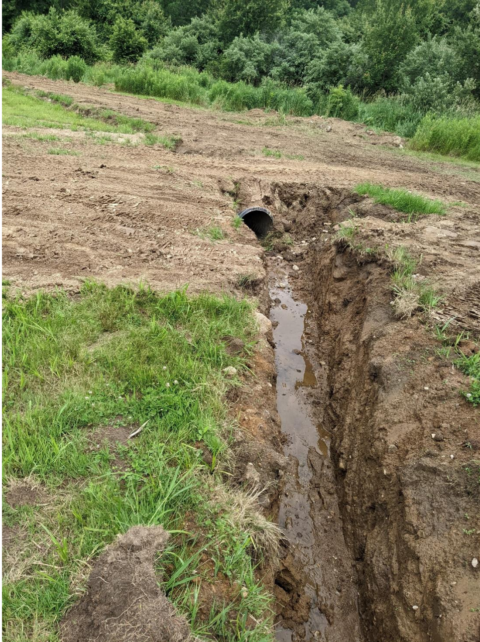
7- View of excavated diversion created by homeowner, looking northwest toward 780 East St. The area in the foreground will remain but will be sloped and graded, with rocks placed in the new streambed to prevent erosion and slow water velocity. The proposed stream will connect this section to the existing stream near the culvert crossing in the photo. This culvert will be relocated upstream closer to the pond, and the remaining area downstream of the culvert will be filled and restored.
