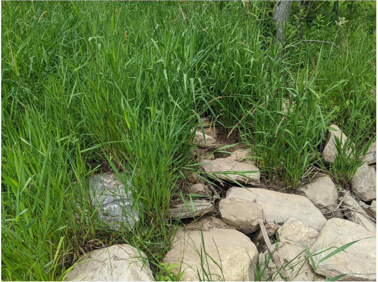
2- View of existing stream channel near pond outlet. Channel is heavily silted and is obstructed by vegetation.
