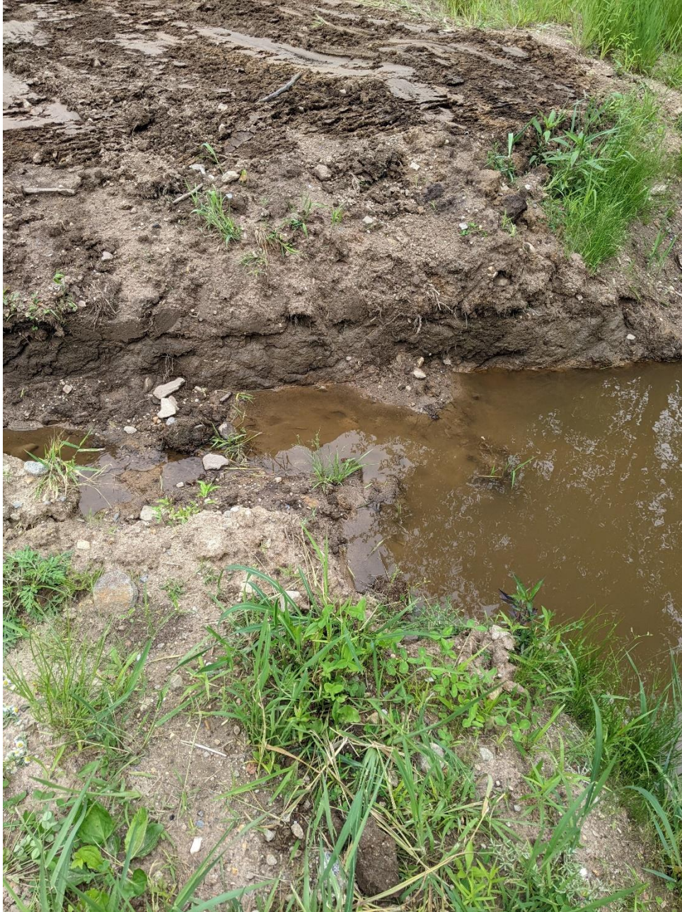
11- View of pond outlet that was created by homeowner. This outlet is proposed to remain, but will be stabilized with rock and graded for erosion control.
