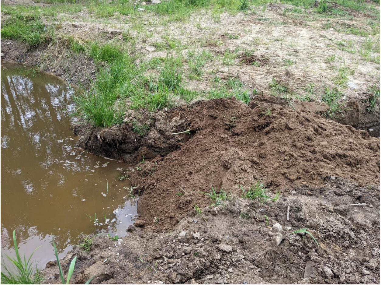
17- Another photo of dam created in the southwestern outlet of the pond (created by homeowner). This dam will remain in place until downstream part of proposed stream is constructed and stabilized.
