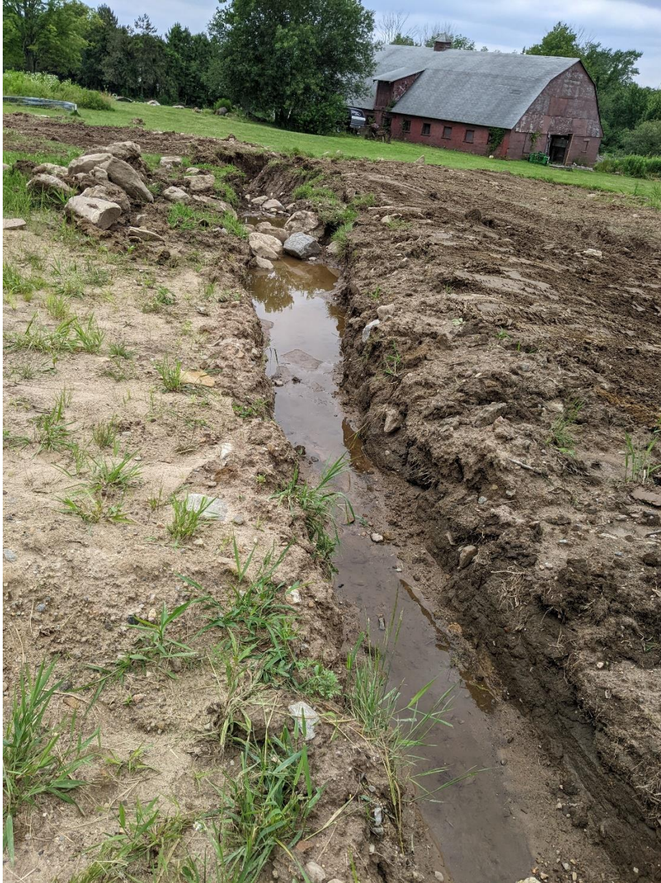
10- View of diversion excavated by homeowner, further downstream than photo #9. This section is proposed to remain in place, with grading and erosion control measures put in place. Proposed pond outlet near western end of pond is behind me.
