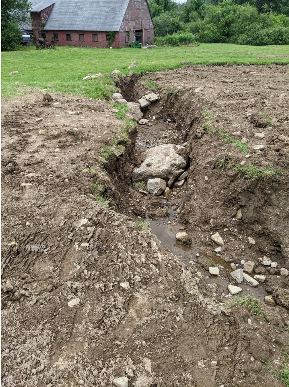
9- View of diversion excavated by homeowner. This section is proposed to remain in place, with grading and erosion control measures put in place. Proposed pond outlet near western end of pond is behind me.
