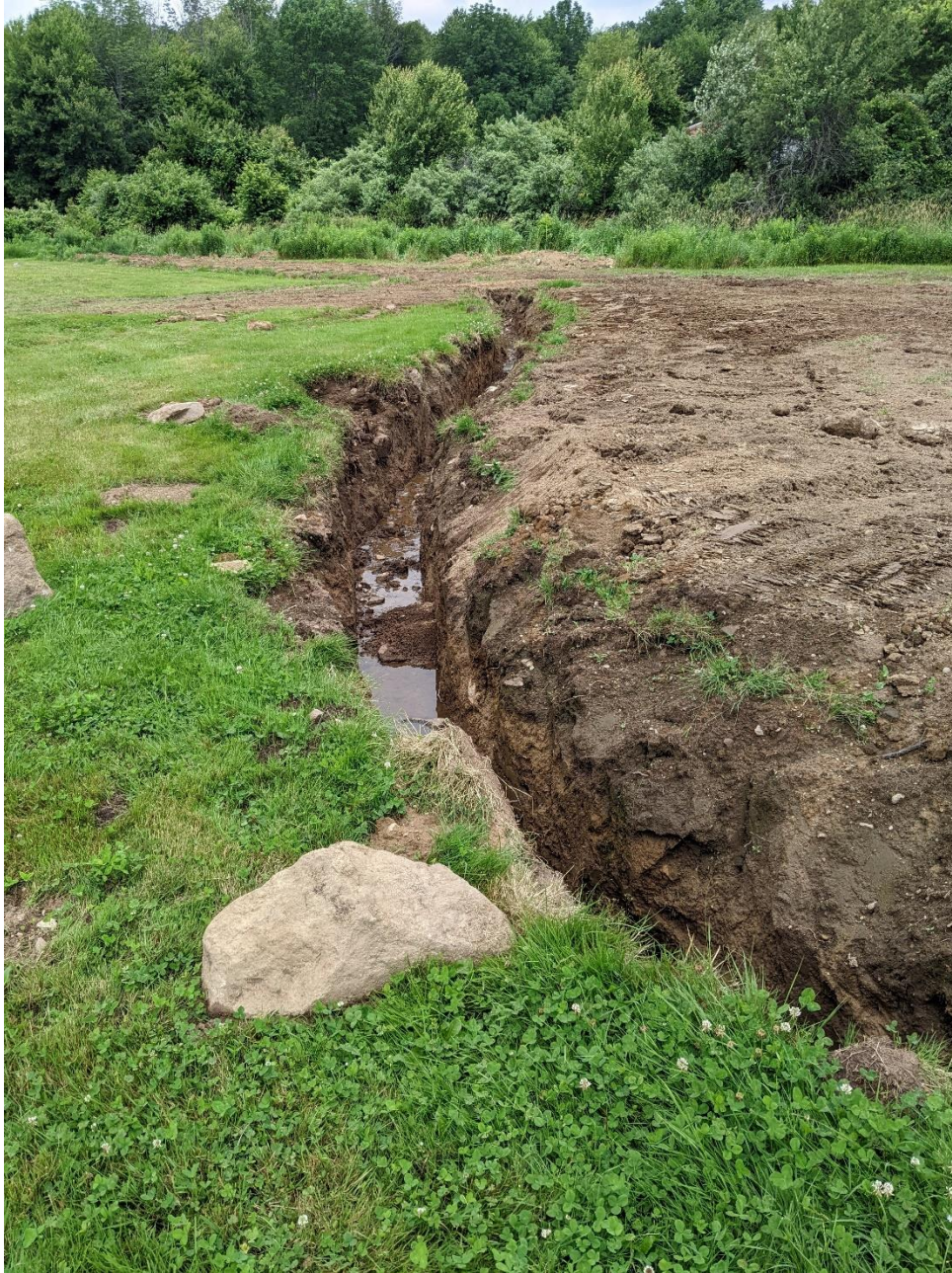
8- View of diversion excavated by homeowner. This section will remain, but will be sloped and stabilized to limit erosion potential. Culvert crossing in center of photo will be closer to foreground to provide access for yard and pond maintenance. Area in top left of photo will be filled and restored.
