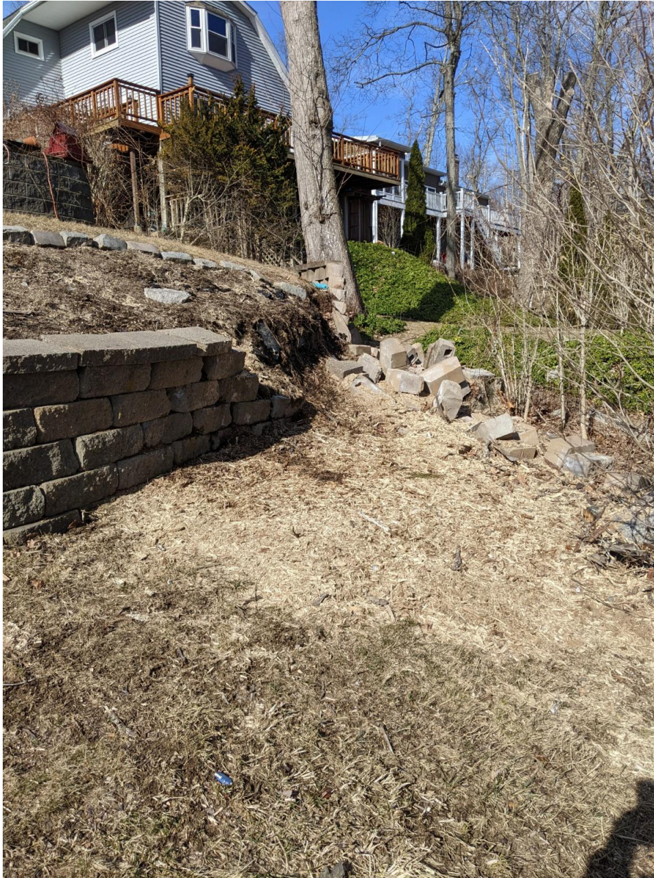
3 View of failed portion of upper wall.
