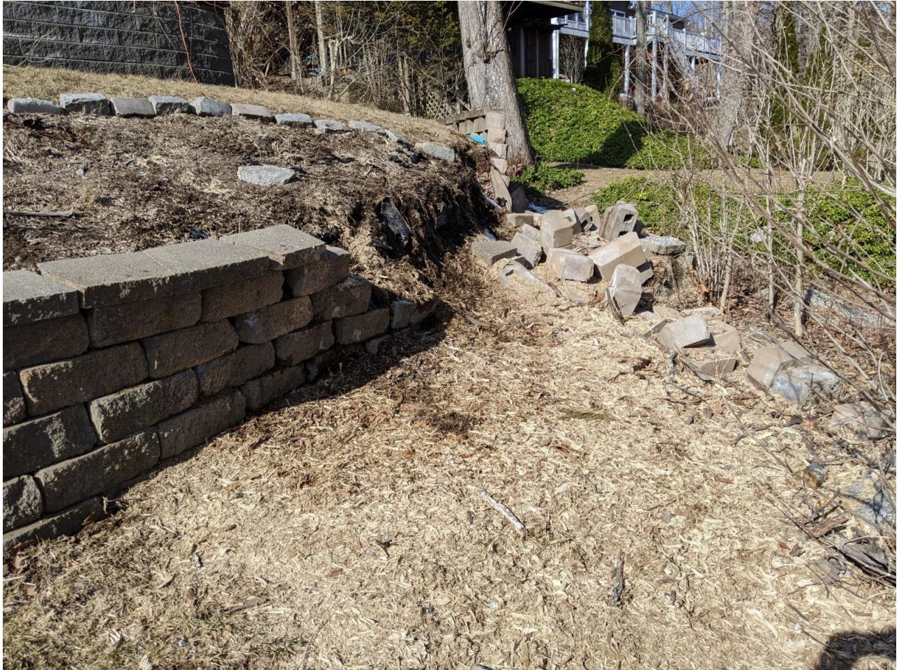
2 View of failed portion of upper wall.
