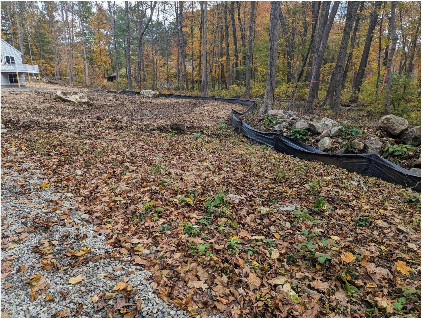
2- View of rain garden, as seen from driveway. Erosion control fencing should be removed when adequate ground cover has been established.
