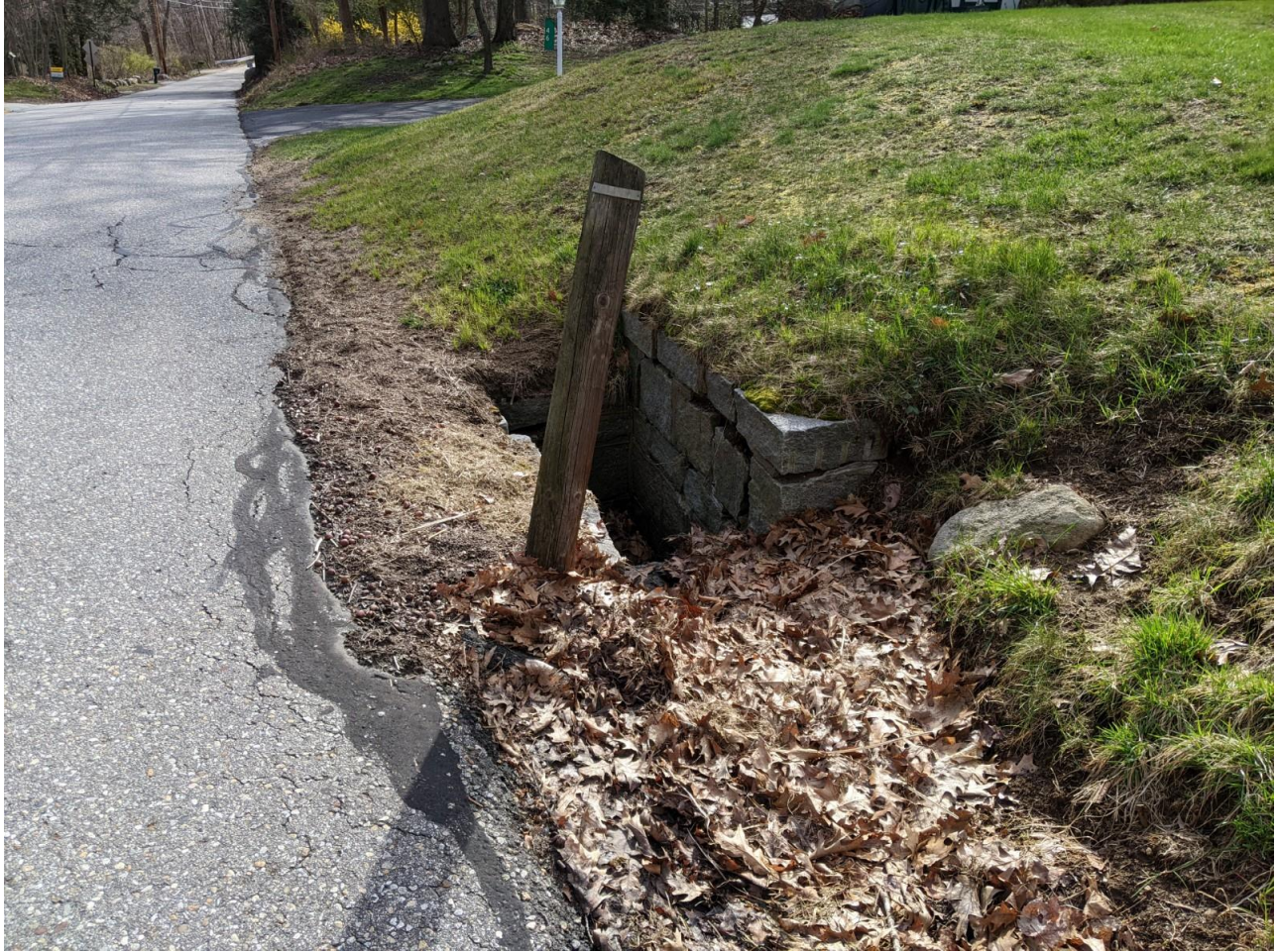
4- View of existing basin on the right-hand (south) side of Shoddy Mill Rd. Pipe runs under the street to the outlet west of 43 Shoddy Mill Road. This pipe and catch basin will be replaced.
