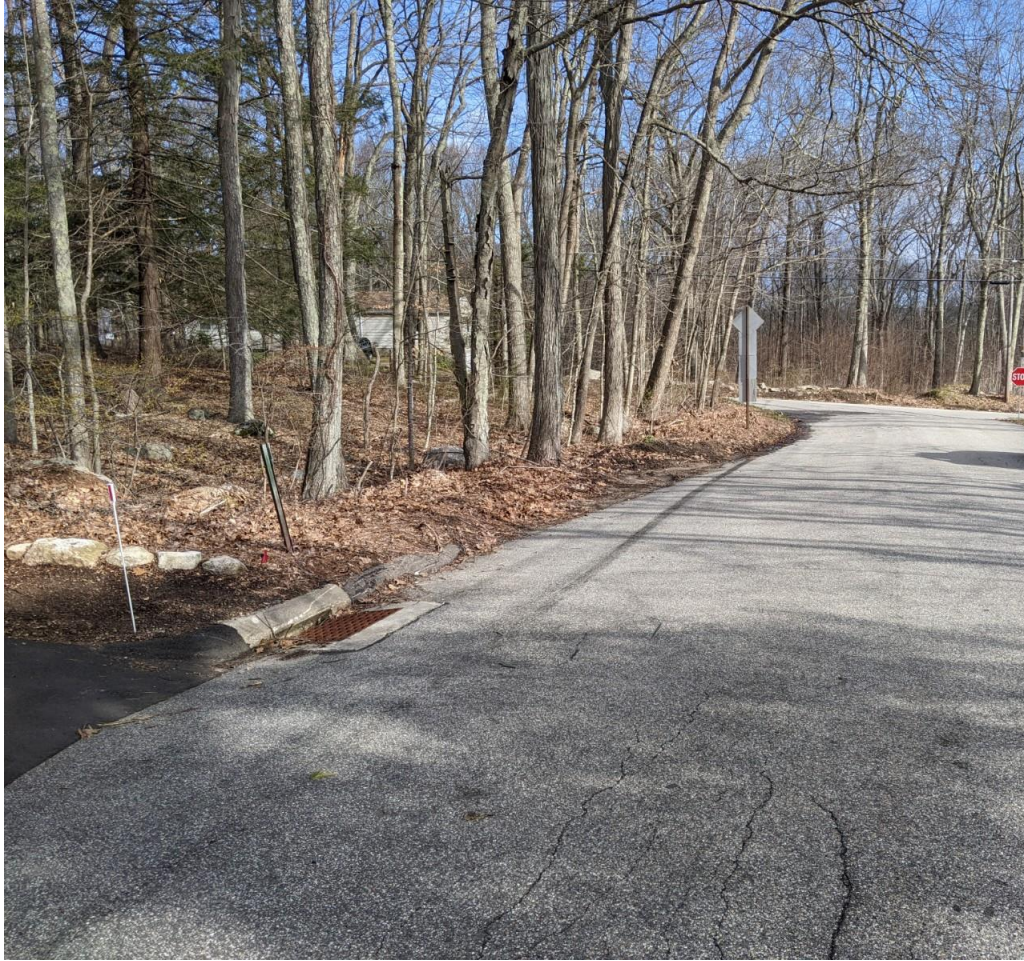
8- View of left-hand side of Birch Drive. Shoddy Mill intersection is in the background. New catch basins, curbing, and piping will be installed in this area to capture runoff that currently flows onto the road.
