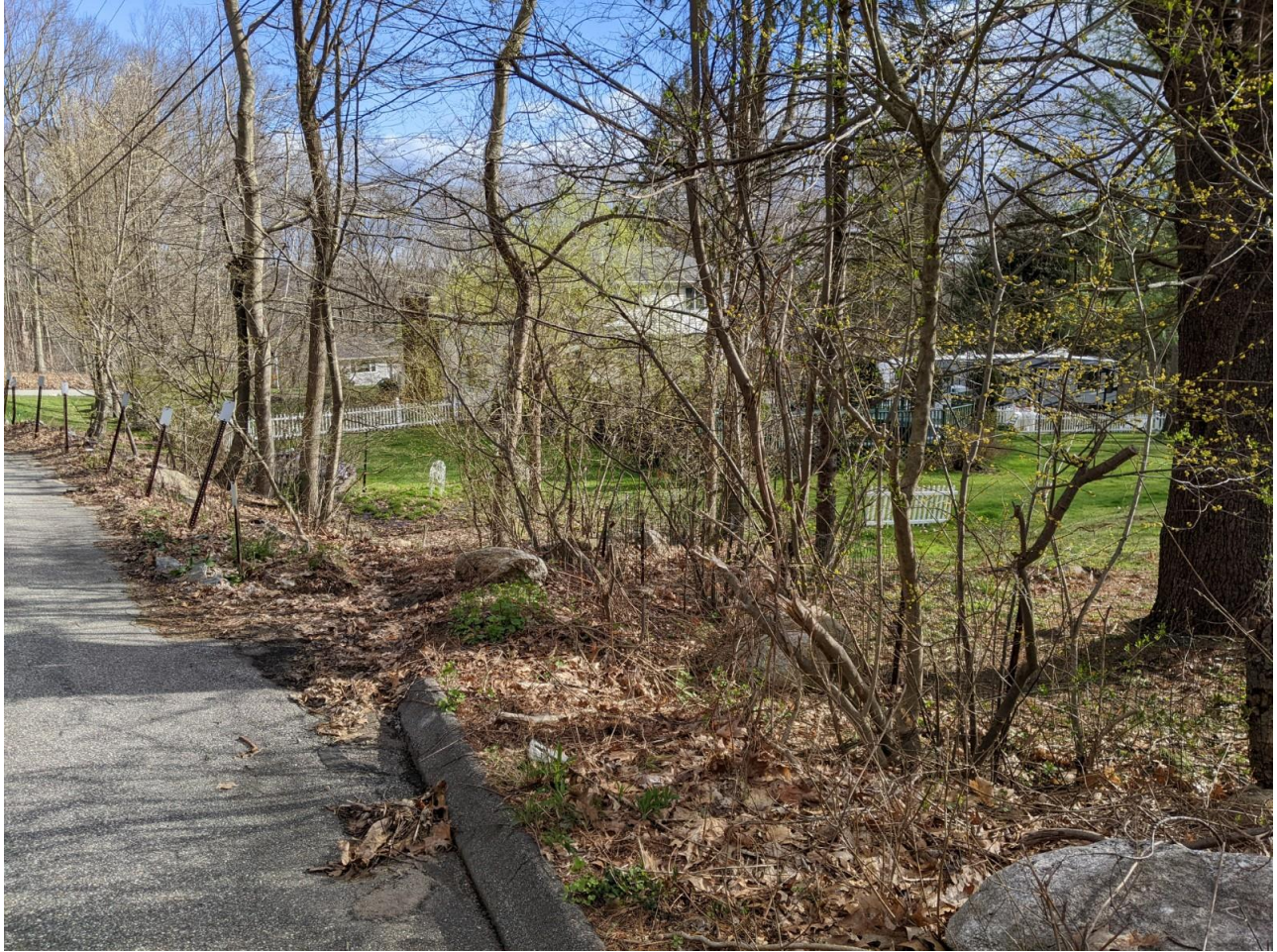
9- View of right-hand side of Birch Dr. 46 Shoddy Mill Rd. is in the top right of the photo. Curbing will be extended to redirect road runoff to the improved storm drains, away from the watercourse and undersized pipe on the 46 Shoddy Mill Rd. property.
