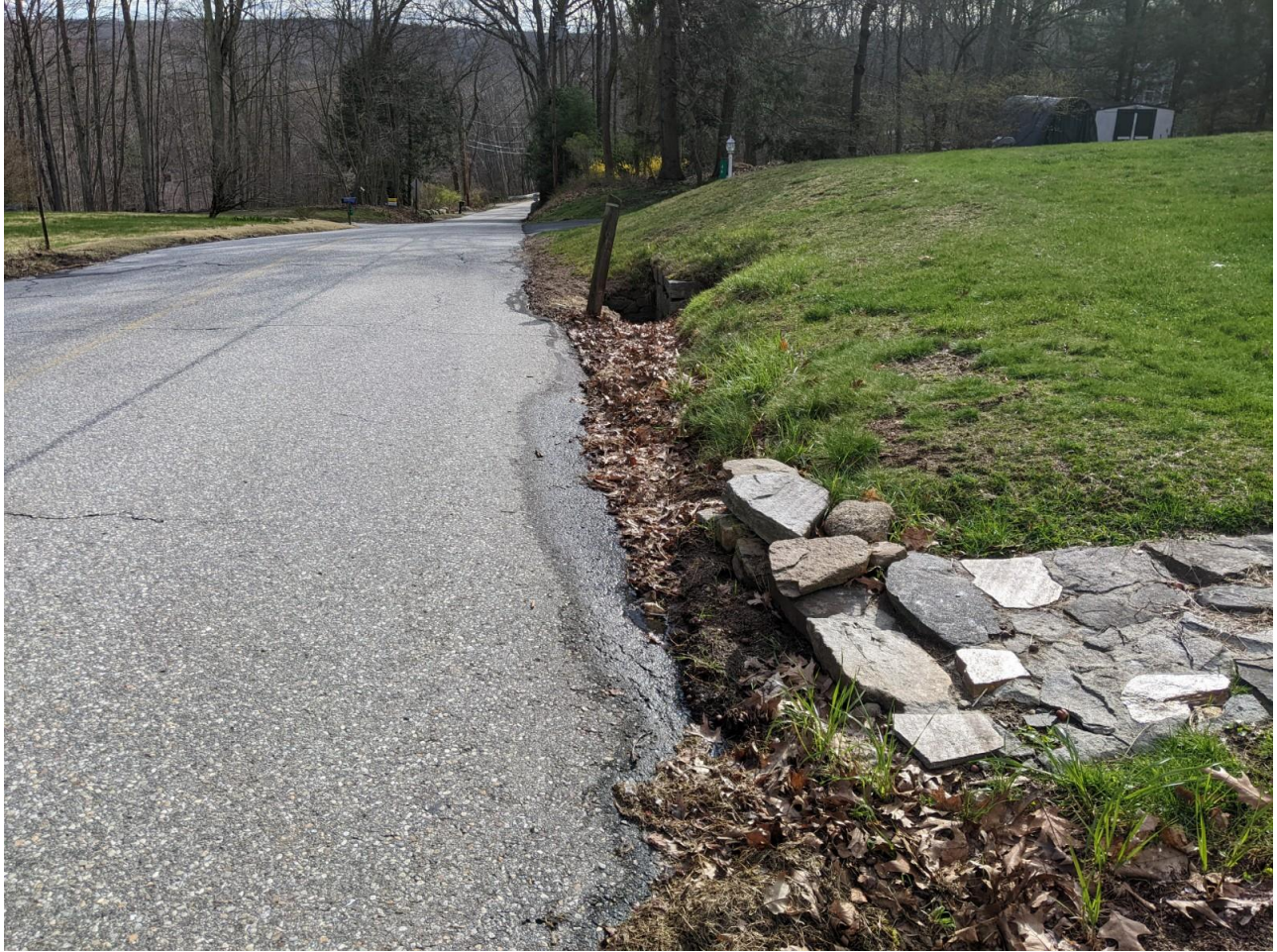
5- View of the right-hand (south) side of Shoddy Mill Rd, looking east. Birch Dr. is behind the photo. Pipe will be installed in this section connecting to a catch basin (the existing basin is in the center of the photo).
