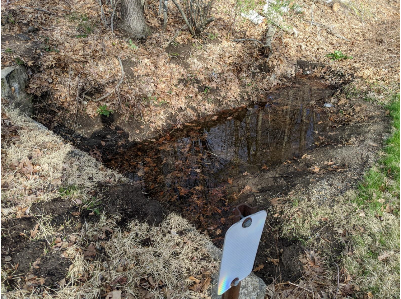
3- Another view of the outlet and watercourse north of 43 Shoddy Mill. Debris and sediment buildup is visible in the top right of the photo--this will be removed to allow better flow.
