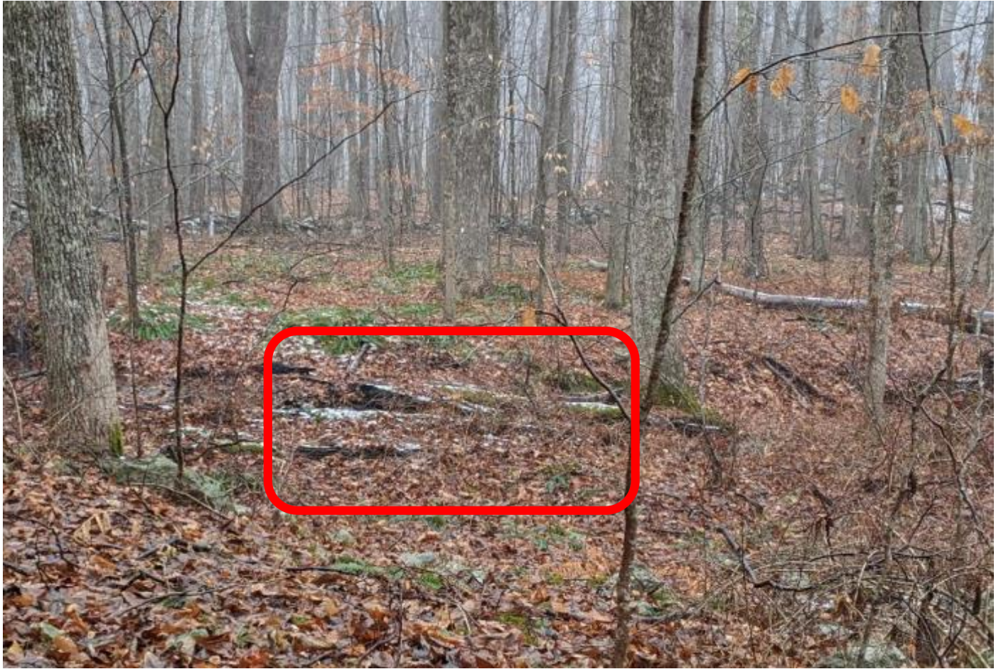
10- View of the approach to the northernmost stream crossing from previous timber harvest. Corduroy used in previous harvest is in the red box.
