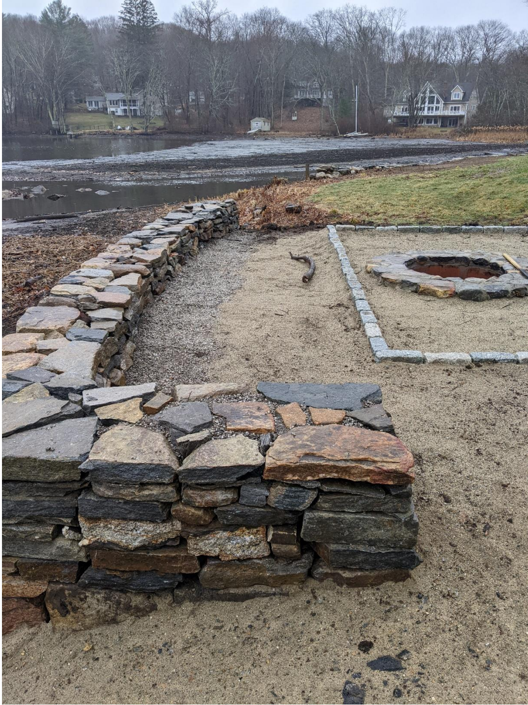
4- View of south wall. There is a 6-foot distance between the fire pit and stone wall. At the recommendation of the contractor, the perched beach outer retaining wall was constructed with "Belgian Block " instead of 4x8 pressure treated posts.
