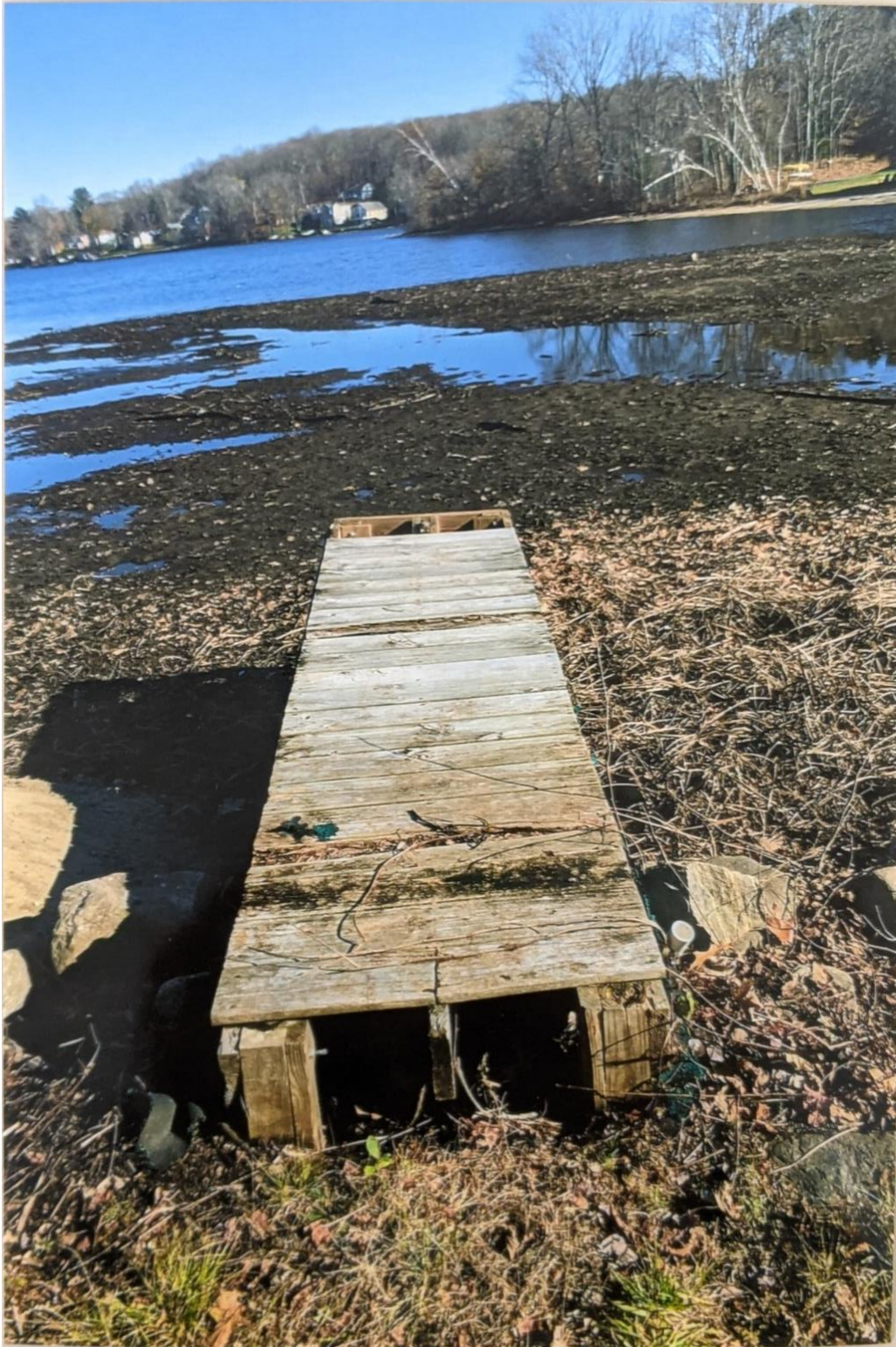
Project #2, Photo #1- View of existing dock. "L" part was deteriorated and has already been removed. Proposed dock will be L-shaped, similar to the existing dock prior to the partial deconstruction.
