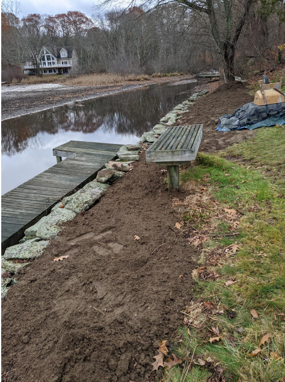
5- View of the center area of the lake wall. This area is proposed to be re-pointed with mortar, but does not need to be restacked.
