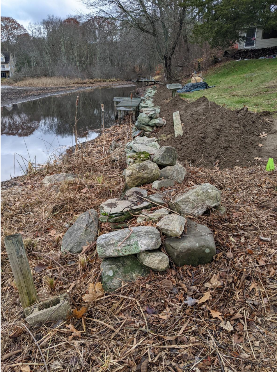
7- Looking along wall from the north end of the property. The crumbled wall in the foreground is proposed to be restacked.
