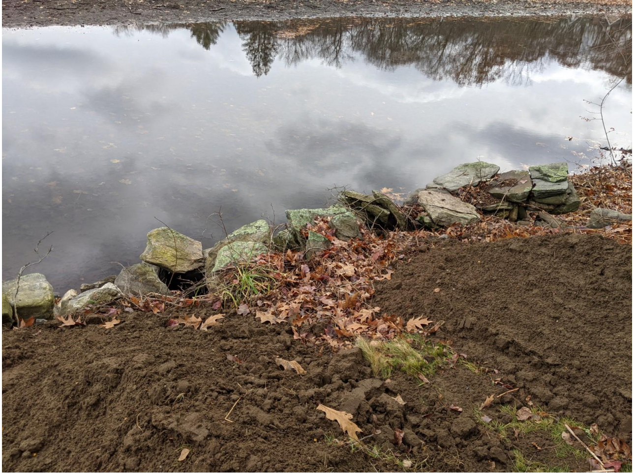
3- Looking down at the southern corner of the lake wall. This end is proposed to be restacked.
