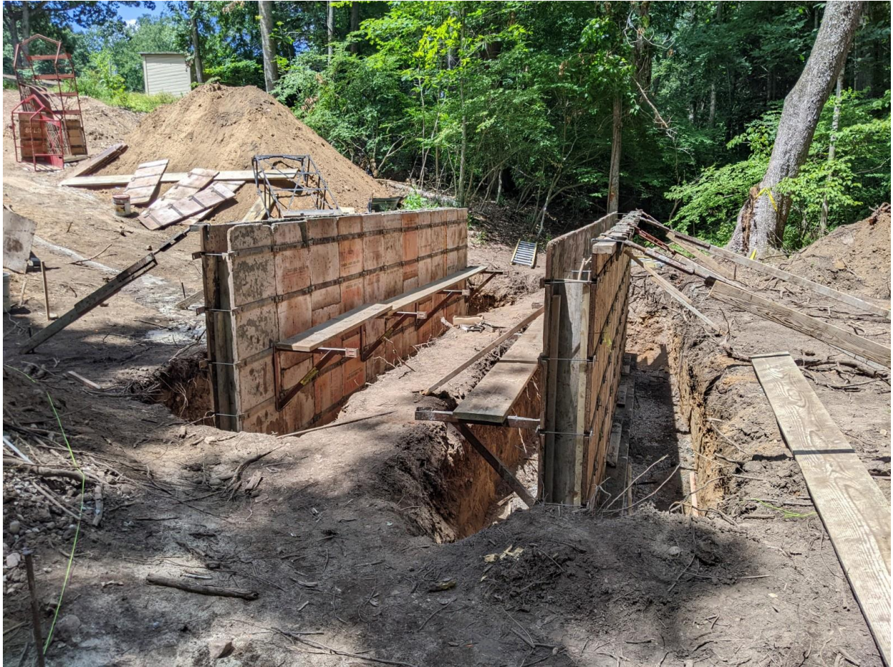
7- View of crossing looking north. Pine ridge drive is to the left of the photo. The center of the stream channel was preserved in order to retain as much undisturbed soil as possible. Taken by Wetlands Agent 07-13-2022.
