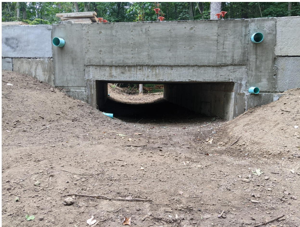
6- Looking north through cast-in-place culvert. Taken by Wetlands Agent 08-22-2022.
