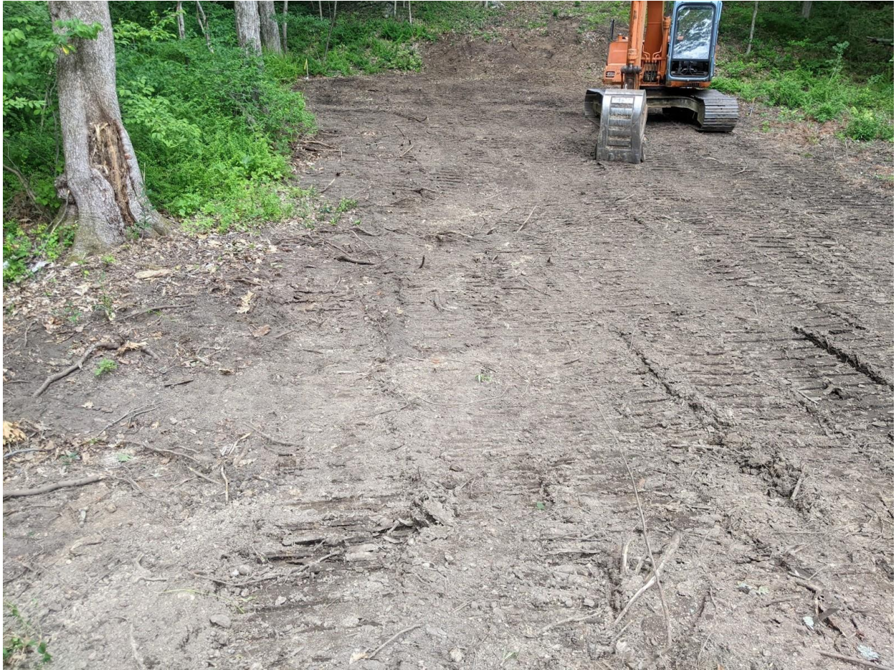
8- View of wetlands crossing site, after clearing and grading and before construction of crossing. Taken by Wetlands Agent 07-06-2022..
