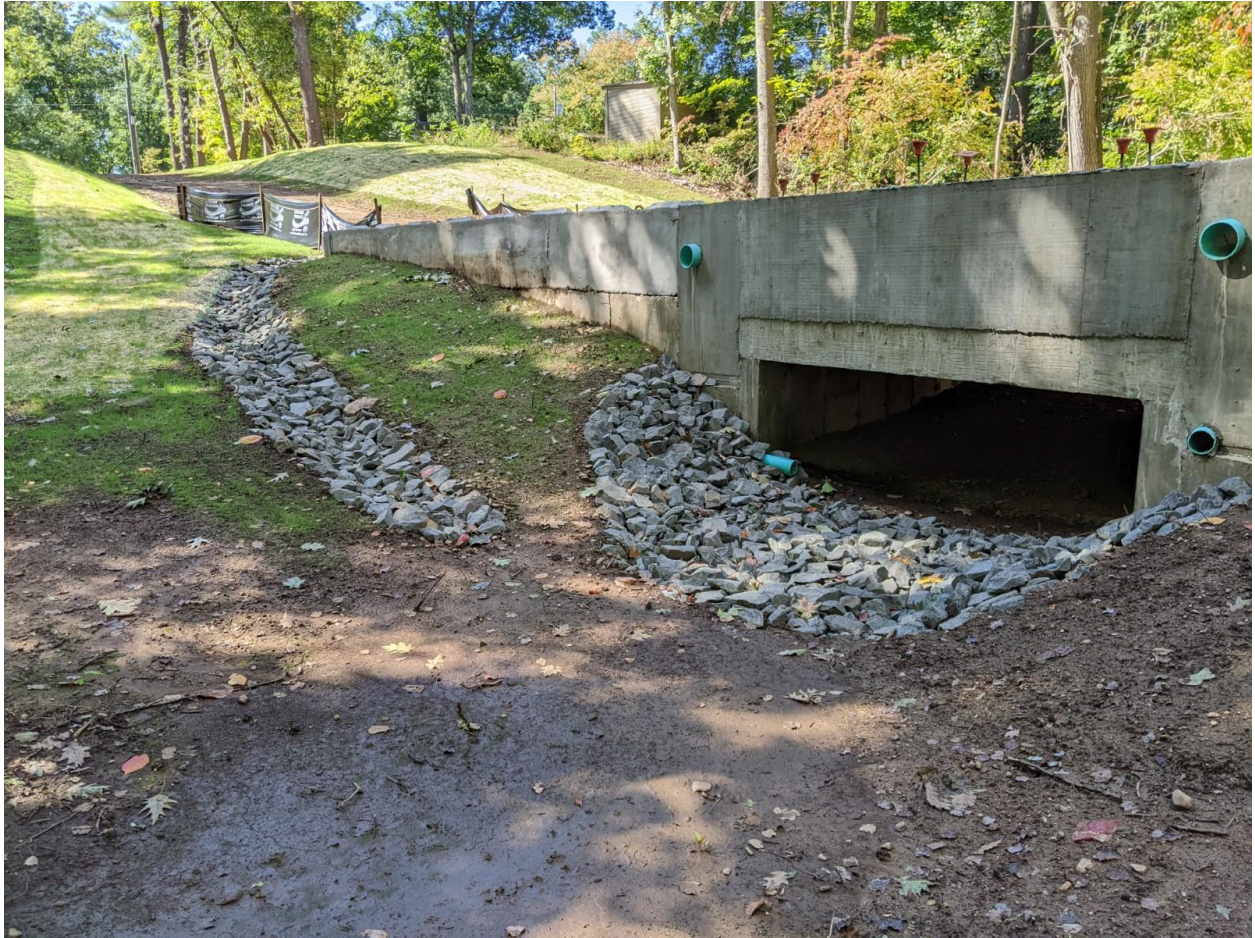
2- View of downstream side of open-bottom culvert. Pine Ridge Drive is toward the upper left corner of the photo. Taken by Wetlands Agent 09-27-2022
