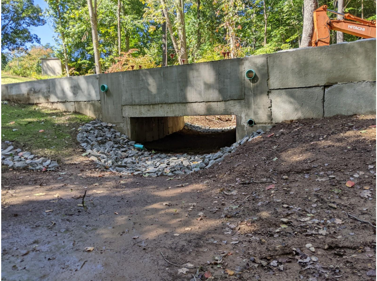
3- View of downstream (southern) side of open bottom culvert. Taken by Wetlands Agent 09-27-2022.
