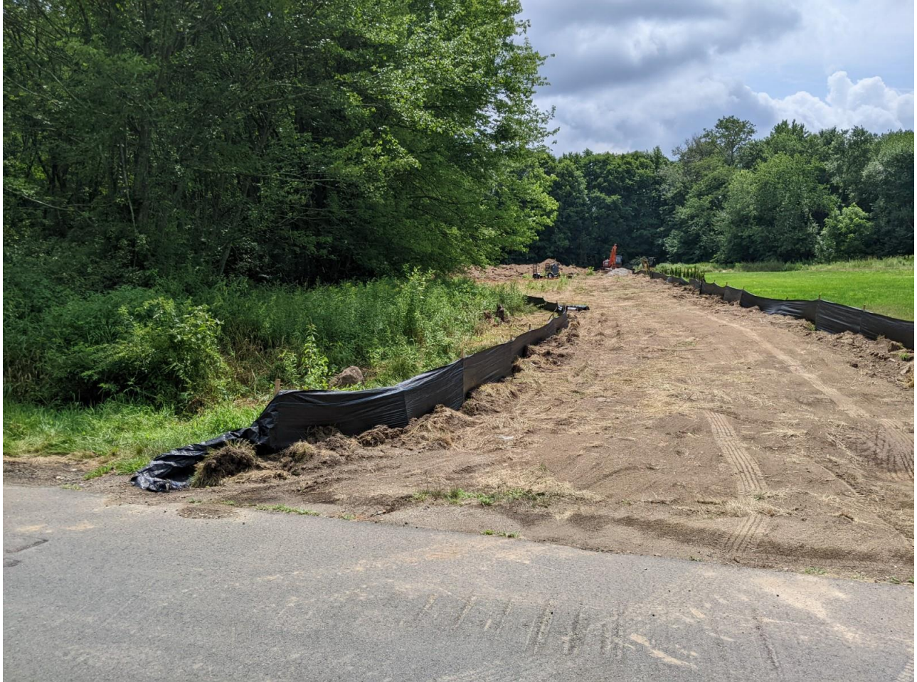
1- View of sediment fence installation, as seen from Webster Lane
