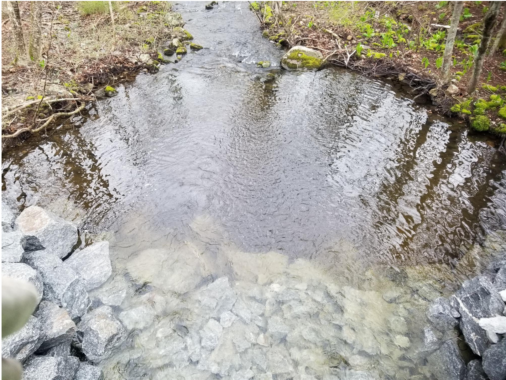
Bunker Hill Rd Culvert (Bear Swamp Brook, TOA) - Pictures after work to protect downstream headwall from erosion and scour. Photos taken by Public Works 04.11.2024
