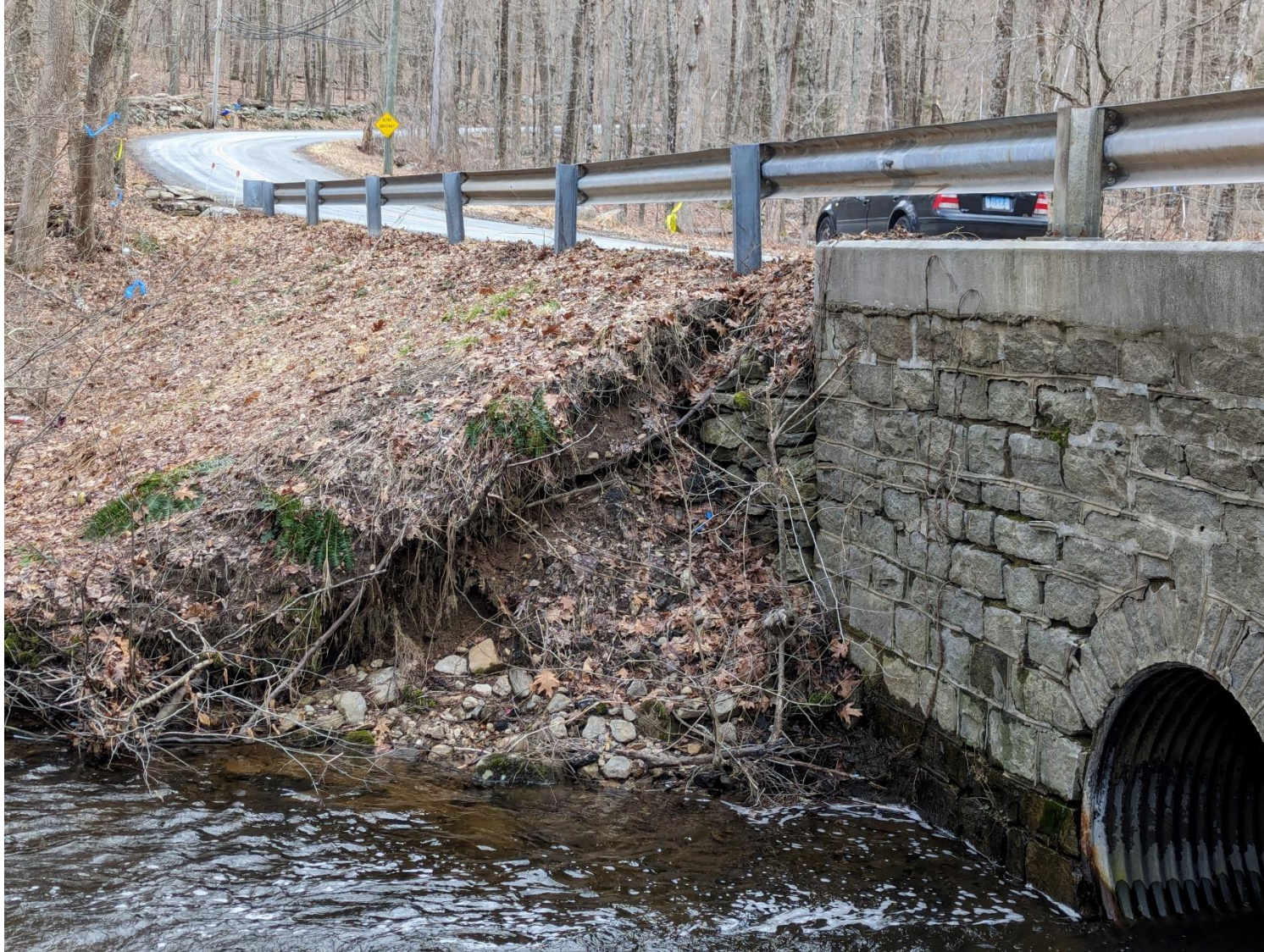
2 - View of downstream side of headwall--erosion is clearly visible.
