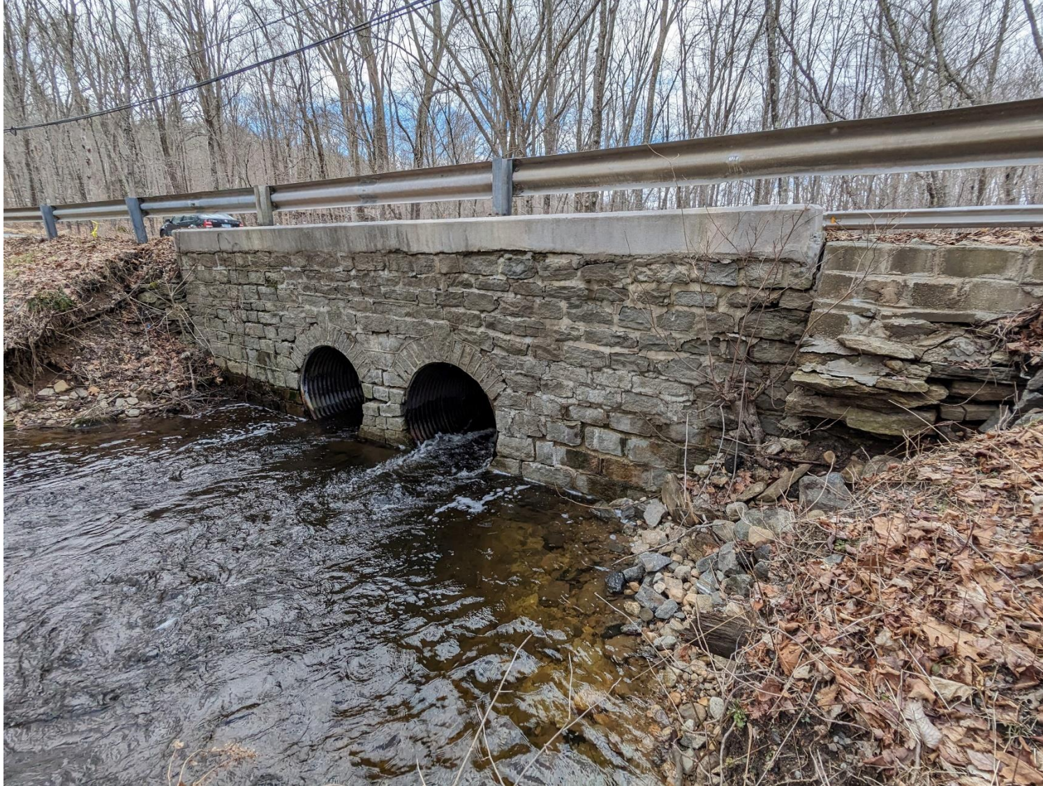
3 - View of downstream side of crossing, where work will take place. Erosion is clearly visible on the sides of the headwall.
