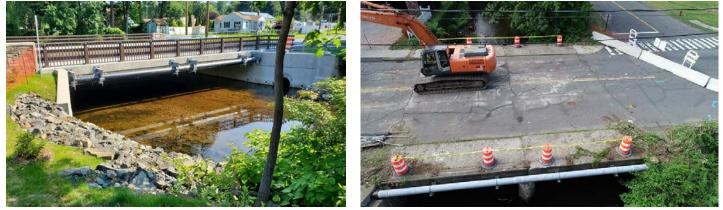
BL Companies provided full-time Construction Engineering & Inspection services for the City of Bristol's Replacement of Bridge No. 04480, the Louisiana Avenue Bridge over Coppermine Brook. The major component of the project was replacement of the existing two-span, 49.5-foot concrete slab superstructure which was supported by concrete abutments and a center pier on spread footings, with a new single-span bridge supported by deep micropile foundations.
